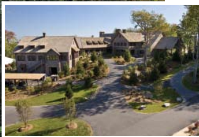
Mountaintop's dramatic par-4 first hole showcases the seasonal colors of the North Carolina highlands. Inset: The recently completed 43,000-square-foot Mountain Lodge. Above right: The crackling fireplace on the Mountain Lodge's cozy porch.
